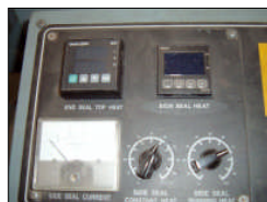
Existing Cabinet Install
